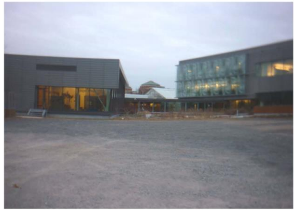
Project construction site
