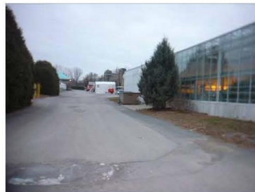
2. Service access road
