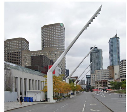
Figure 22 : superstructure-type lampposts in the public spaces
