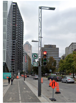
Figure 21 : practical street lamppost
