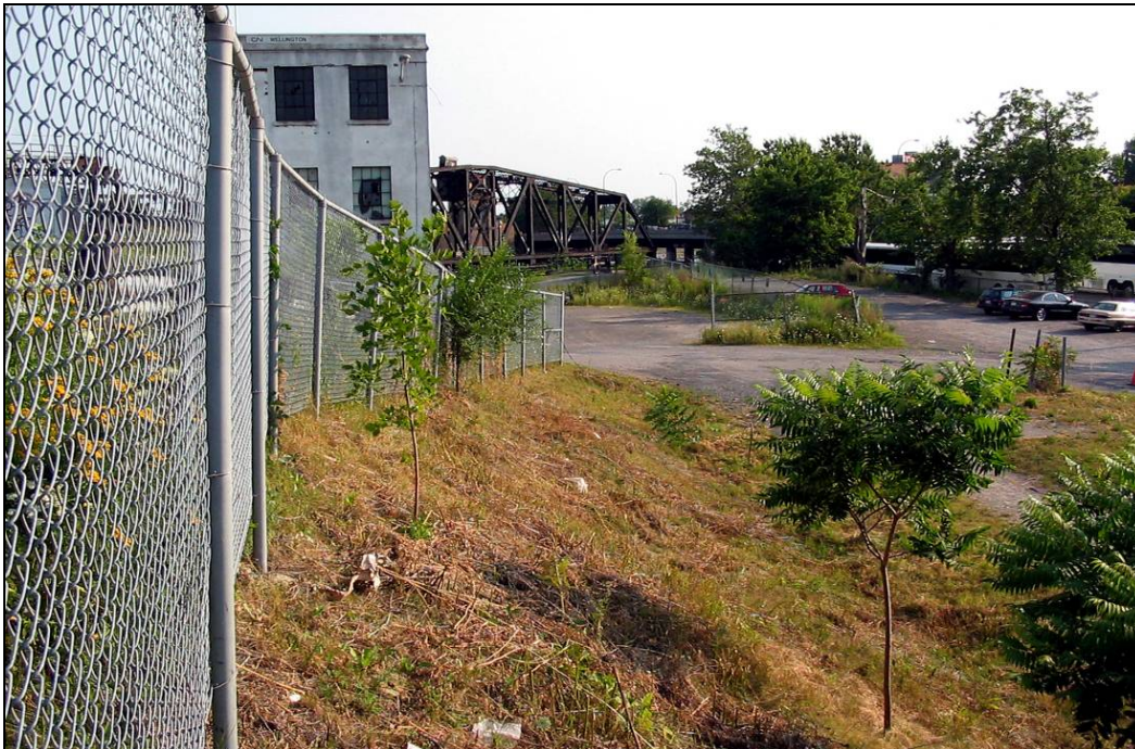
FIGURE 9: VIEW OF SMITH STREET AND THE SWING BRIDGE FROM THE TOP OF THE RAILWAY EMBANKMENT.
