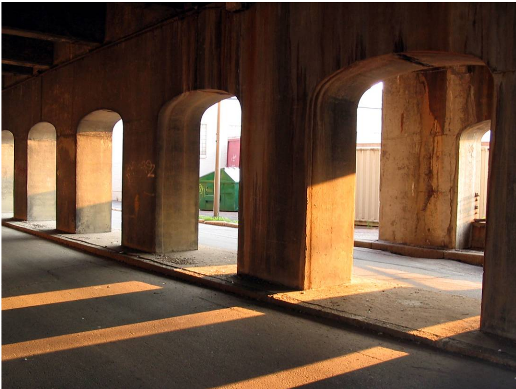
FIGURE 5: UNDER THE CN VIADUCT ARCADES
