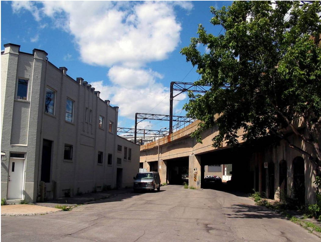
FIGURE 4: PASSING UNDER THE CN, SEEN FROM THE SHANNON STREET INTERSECTION
