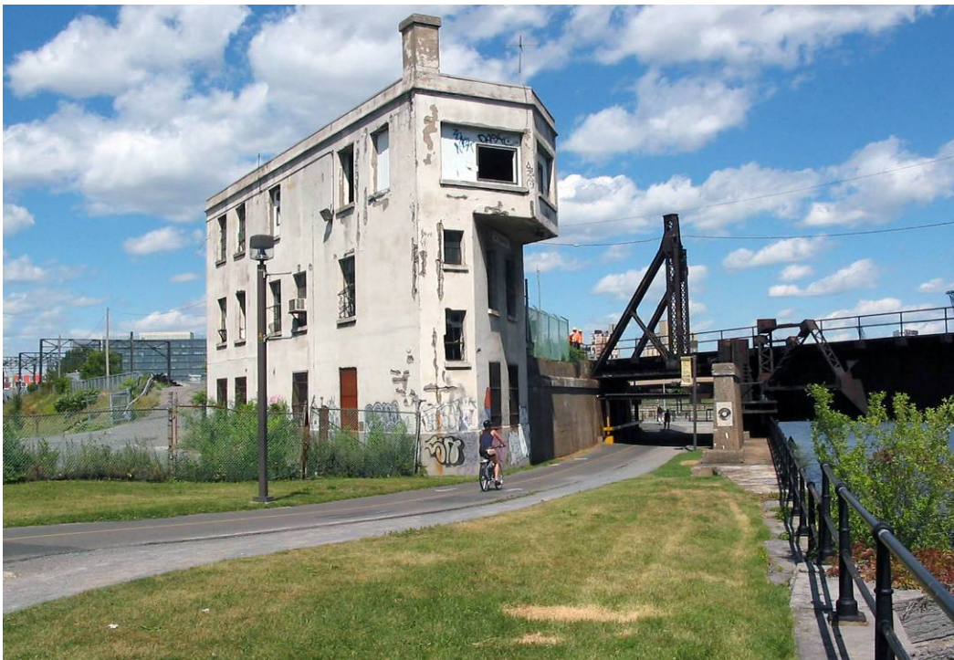
FIGURE 10: FORMER CN SWITCHING TOWER
