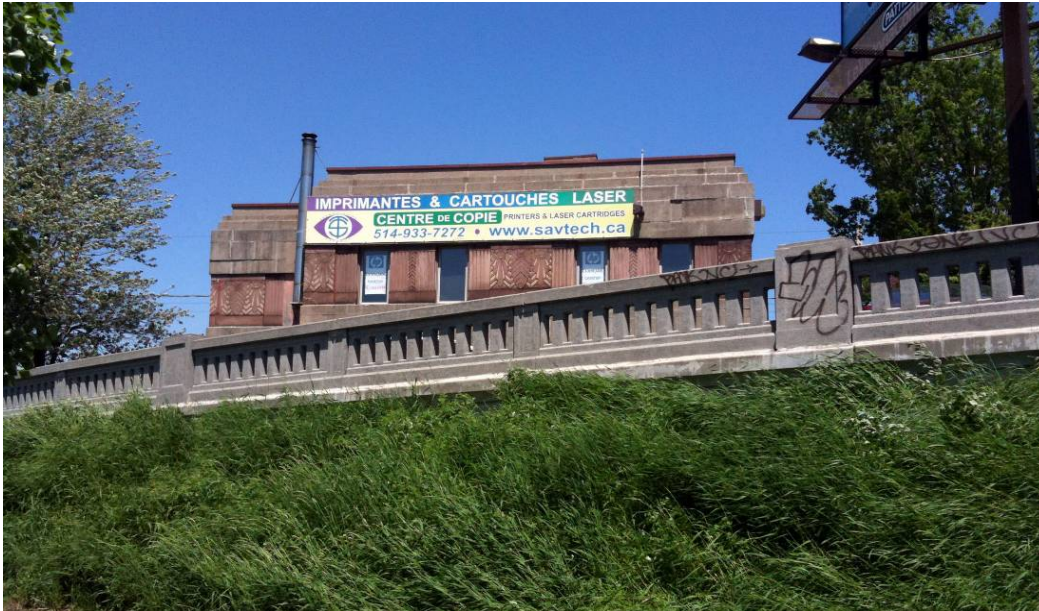
FIGURE 11: FORMER SQUARE GALLERY COTTAGE, SEEN FROM THE WELLINGTON TUNNEL ENTRANCE.
