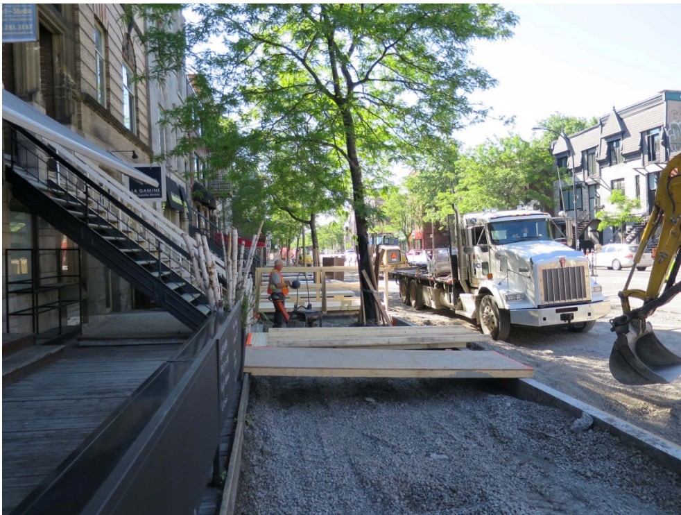
Work on sidewalks; pedestrians redirected to the centre of the roadway
