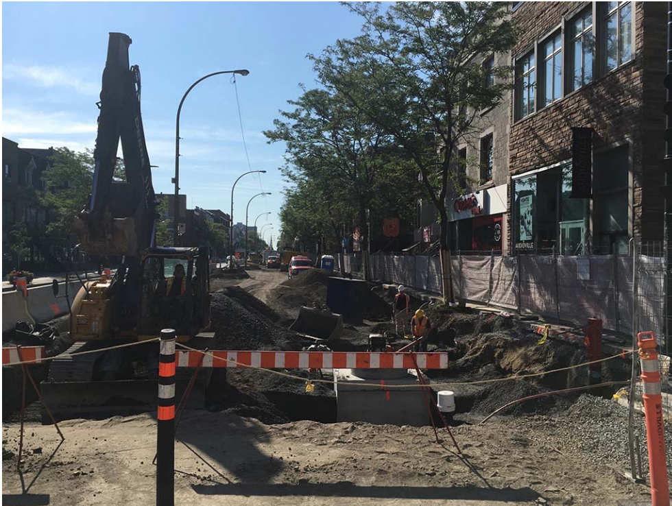
Work on the roadway; pedestrians redirected to the sidewalks
